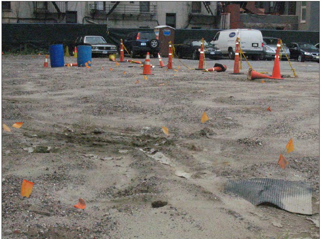
View facing toward the south corner of the project site 3
