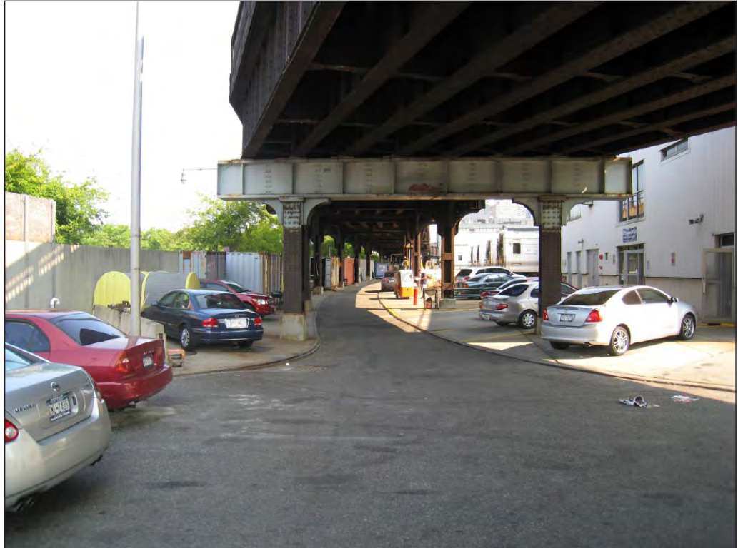
View facing northeast from underneath the High Line 11
