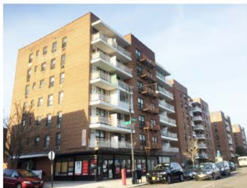
Seven-story apartment building on eastern end
