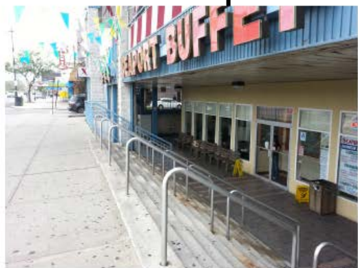
Below grade retail space in cellar
