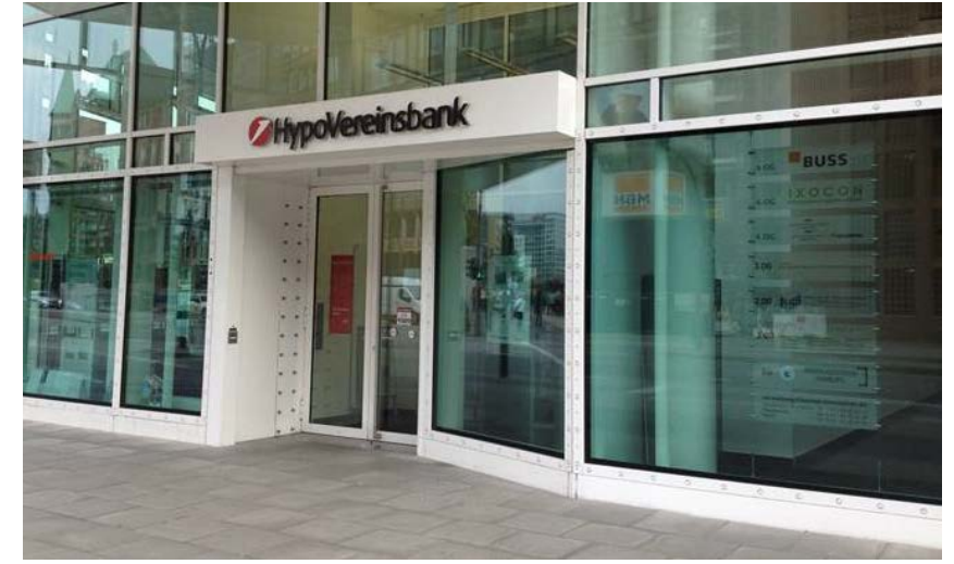
Integrated floodproofing (‘aquarium-grade’ glass for glazing or curtain-wall systems)
