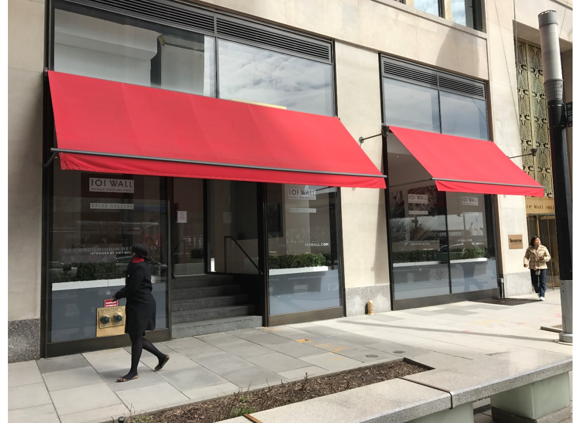
Commercial Building elevated to DFE
