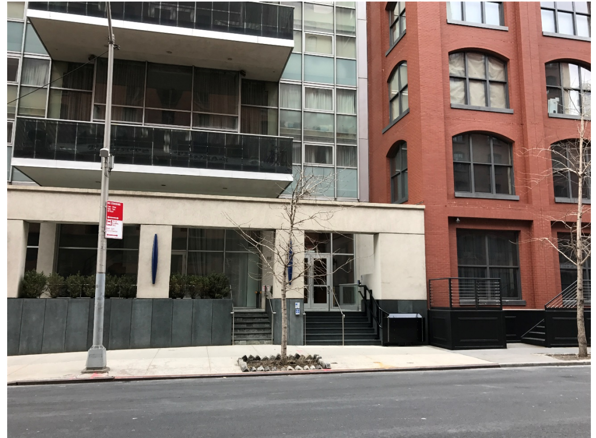
Residential Building elevated to DFE
