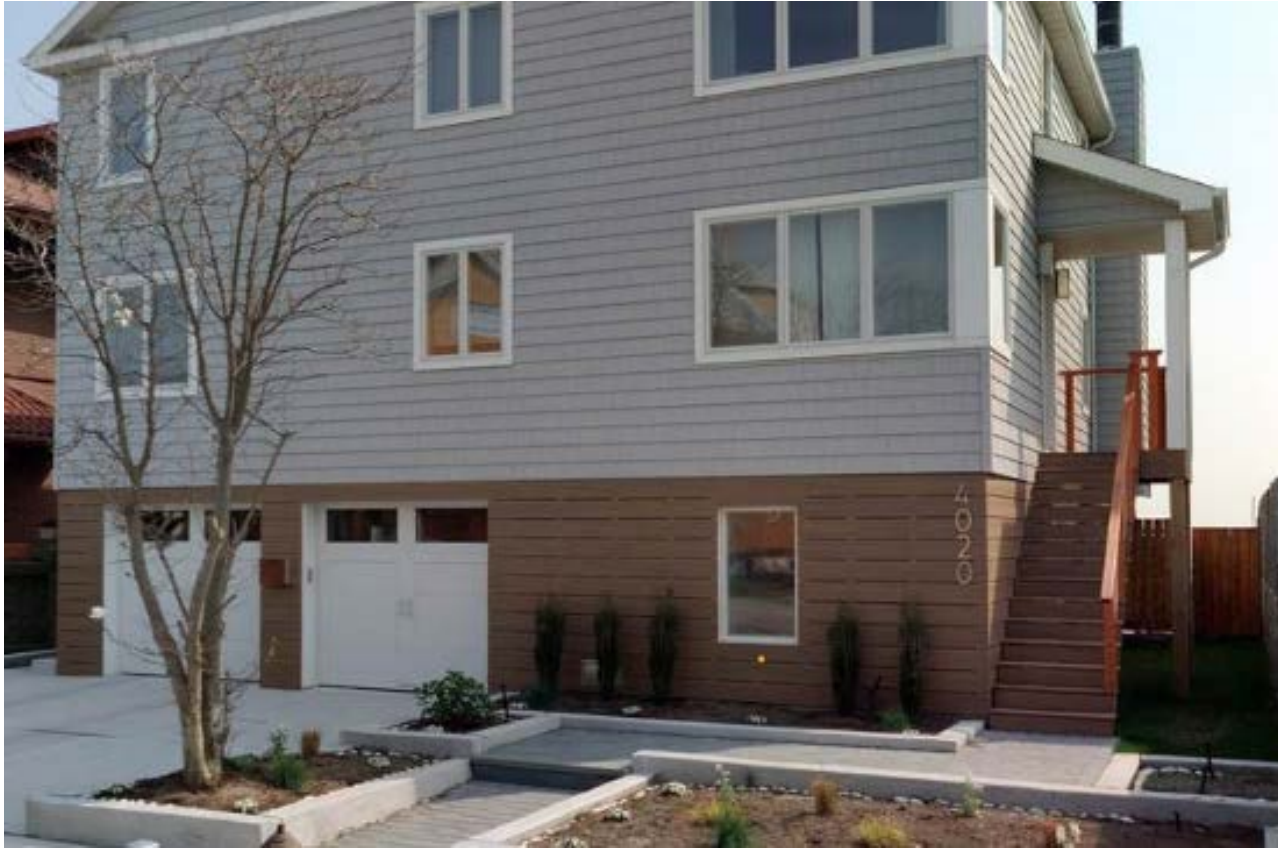
Residential Building Elevated to DFE
