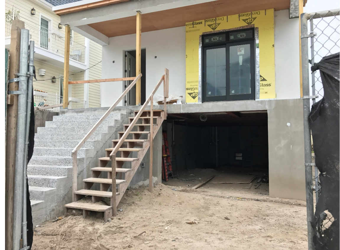
Residential Building Under Construction Elevated to DFE
