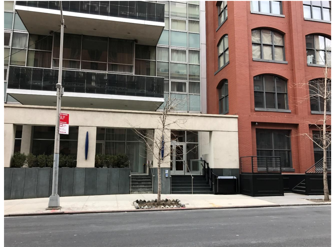
Residential Building Elevated to DFE – 3' above grade
