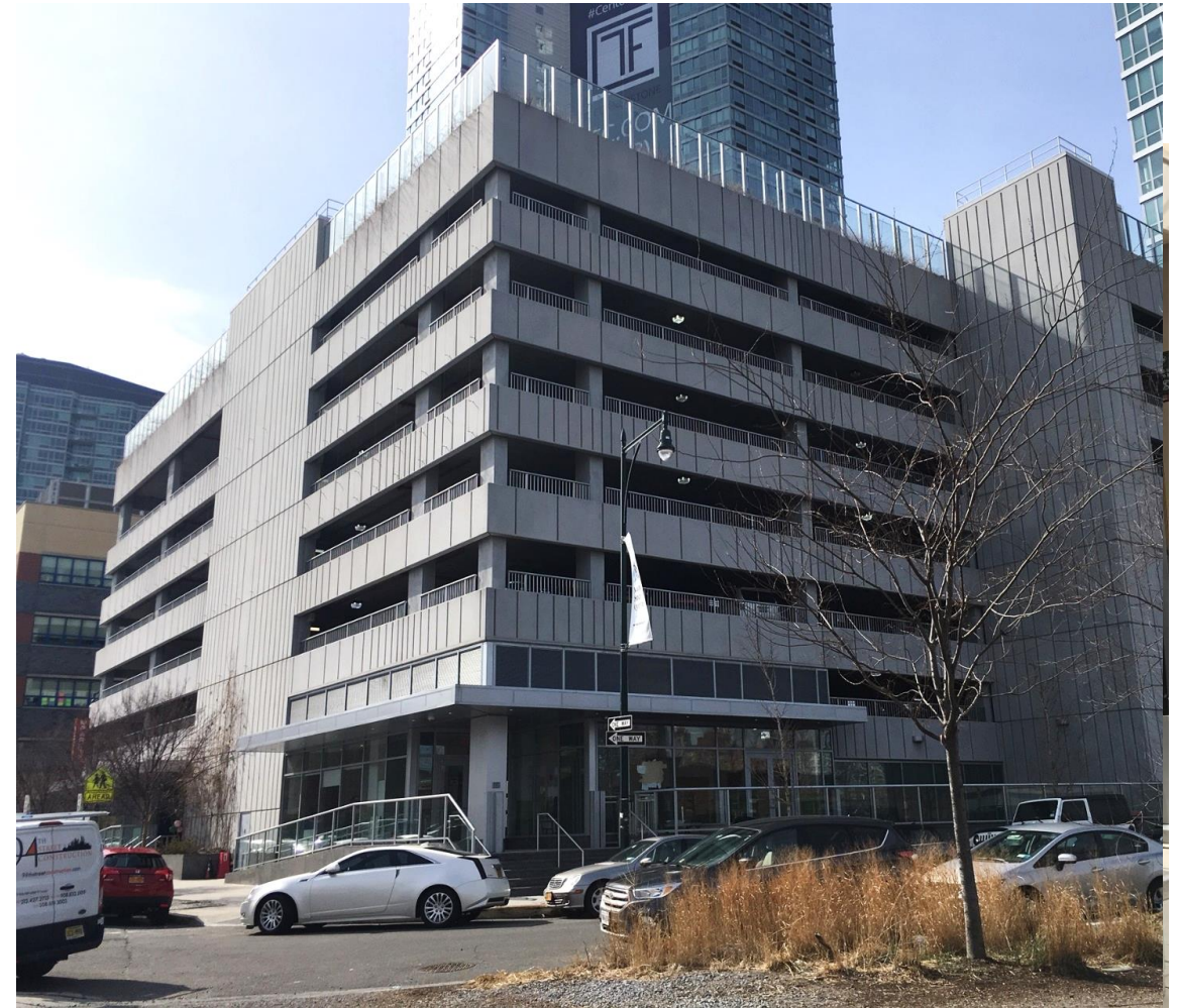
Commercial Ground Floor Elevated to DFE – 2.5'
