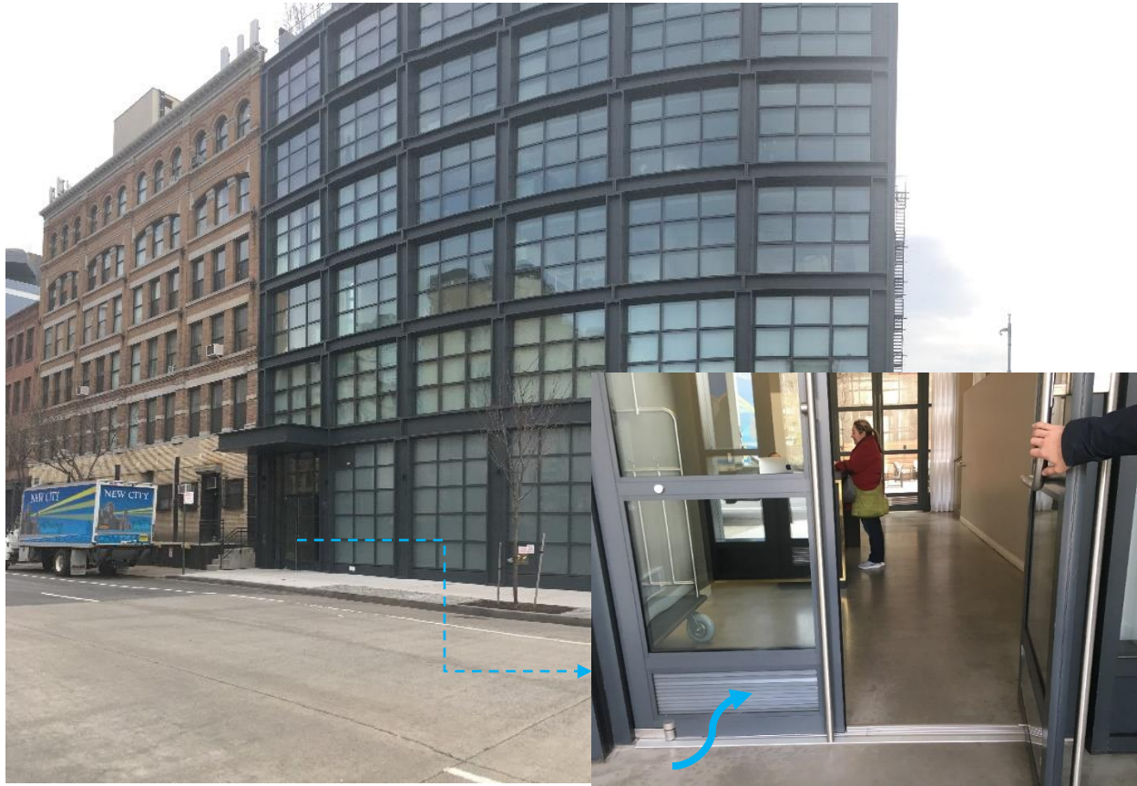
Residential Building with access at grade (wet-floodproofed)
