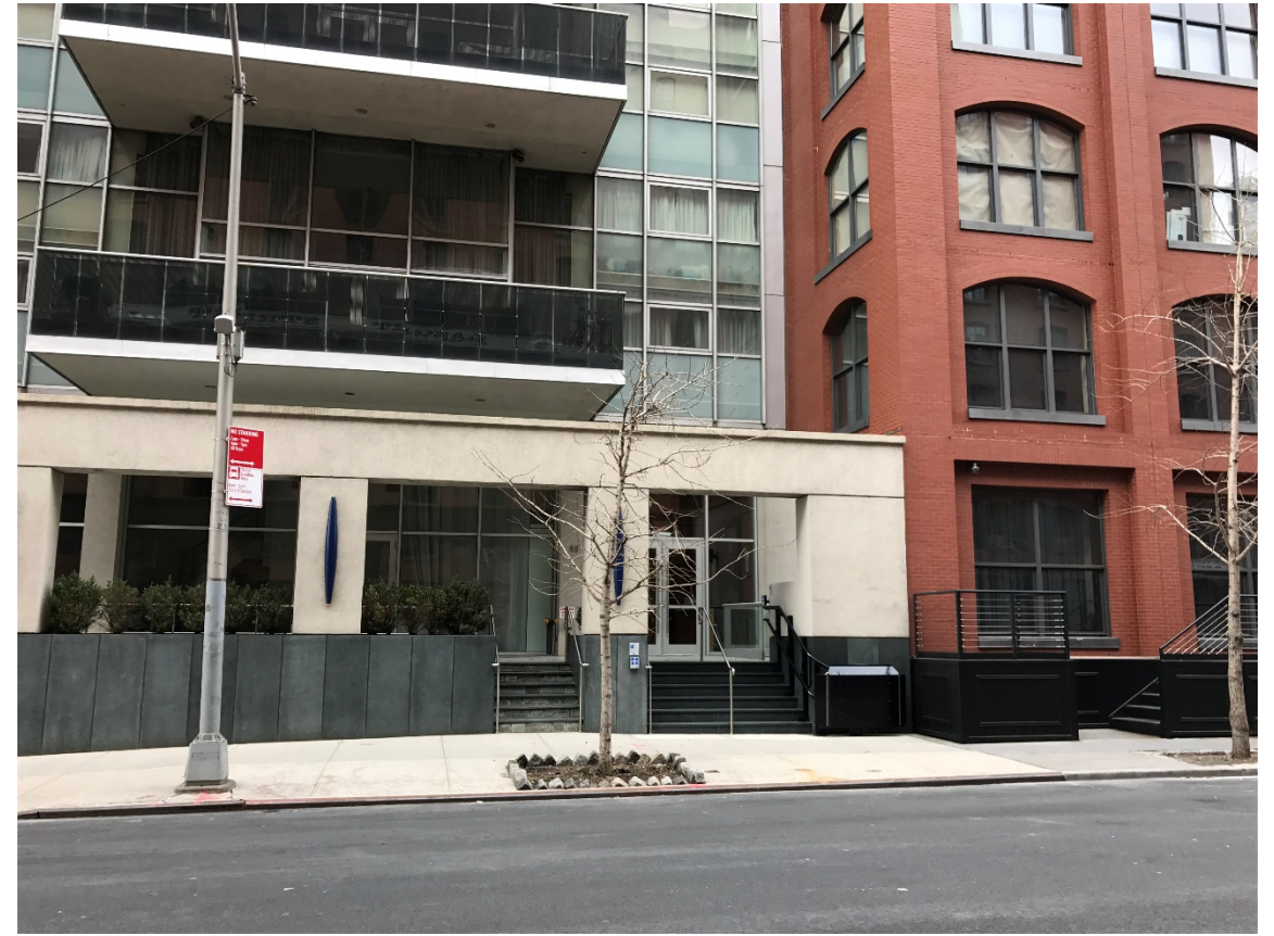
Residential Building in Manhattan Elevated to DFE (~3' above grade)
