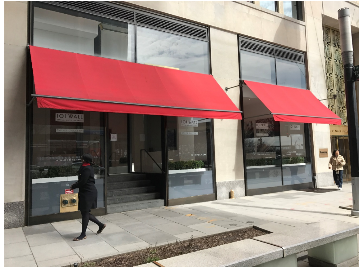
Commercial Ground Floor in Manhattan Elevated to DFE (~2.5' above grade)
