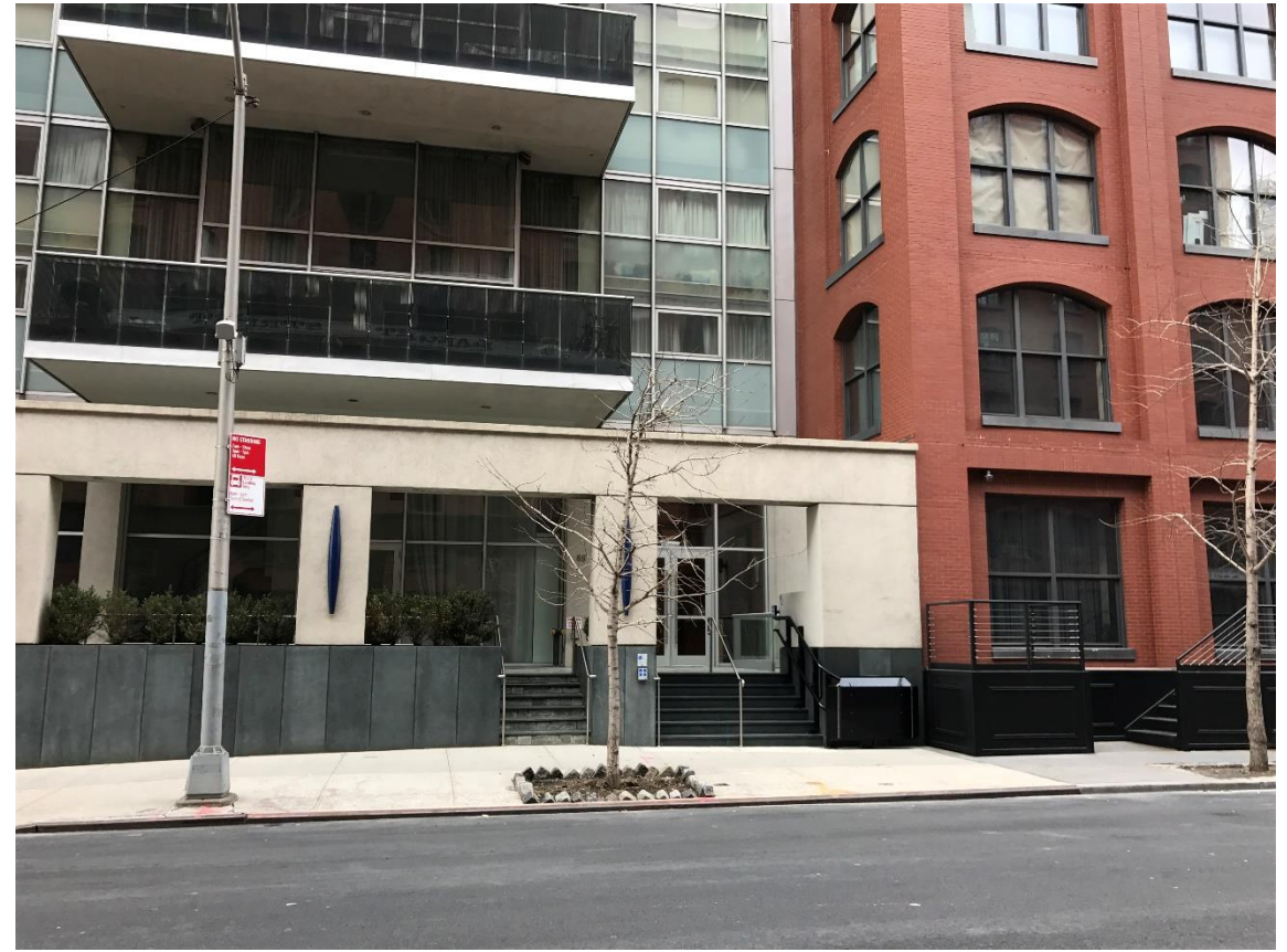
Residential Building Elevated to DFE – 3' above grade
