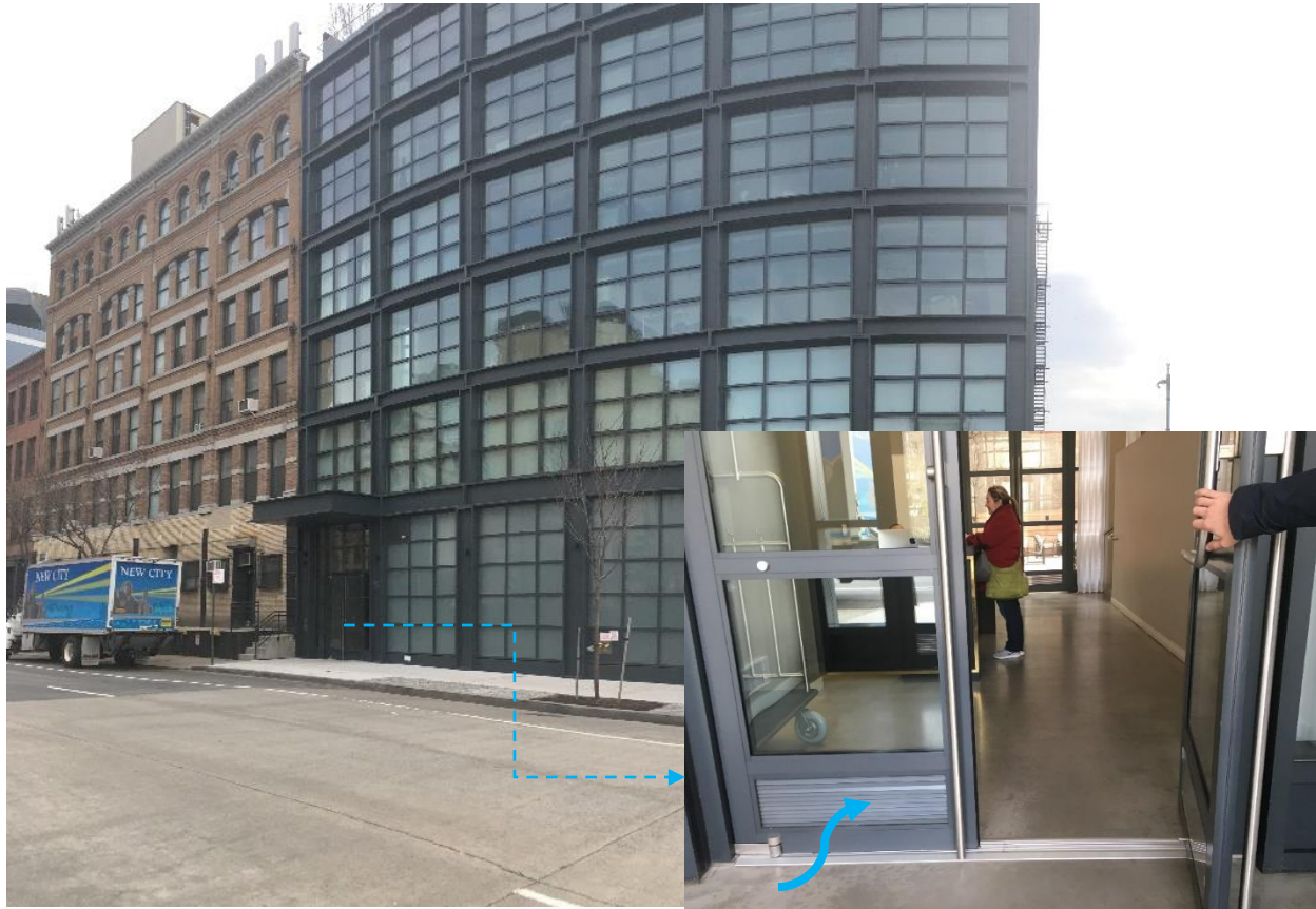
Residential Building with access at grade (wet-floodproofed)
