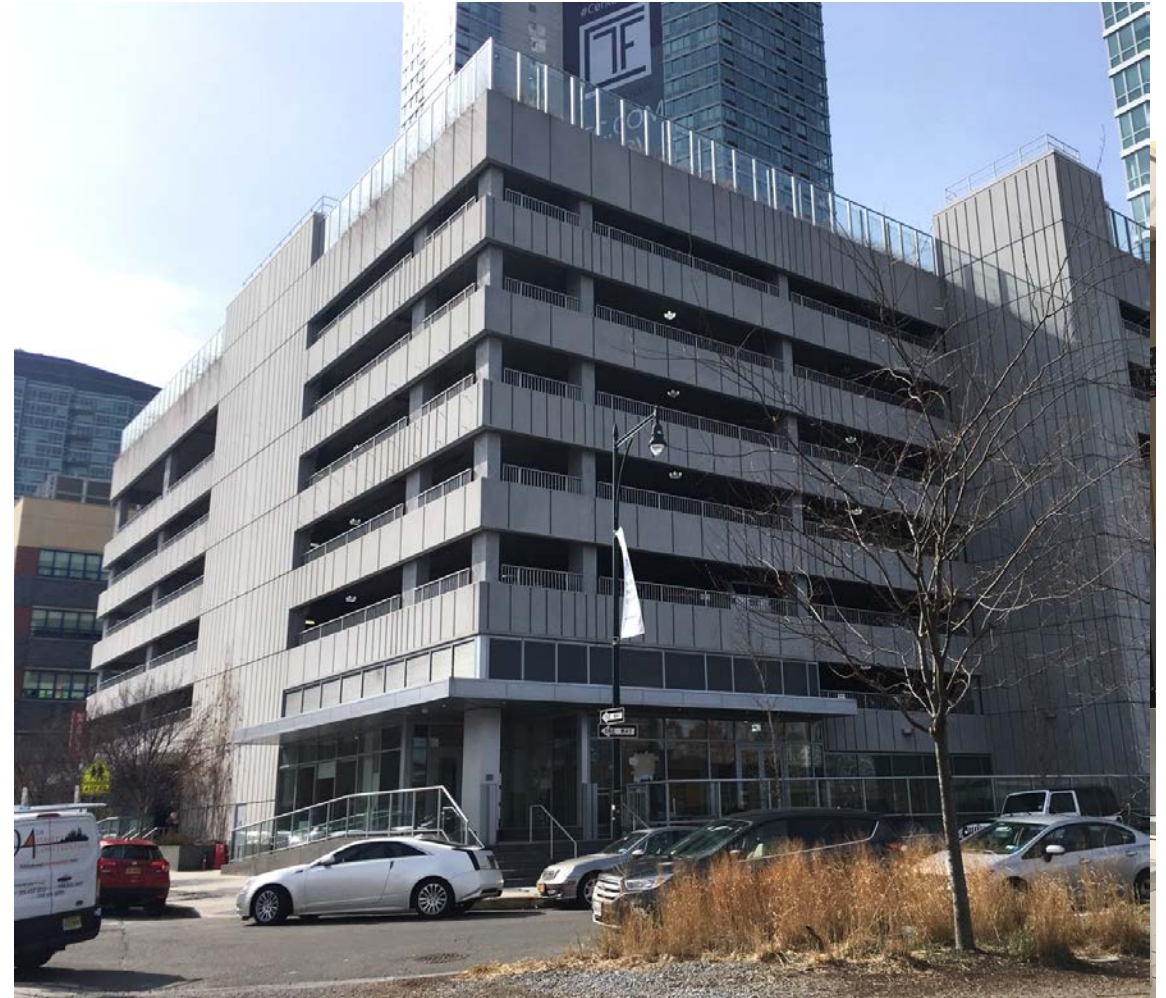
Commercial Ground Floor Elevated to DFE – 2.5'
