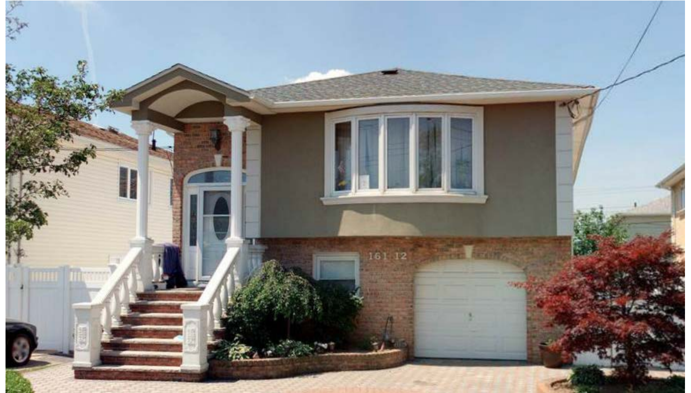
Resilient Residential Building – Elevated to DFE
