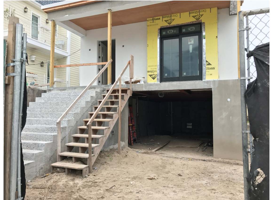
Residential Building Under Construction Elevated to DFE
