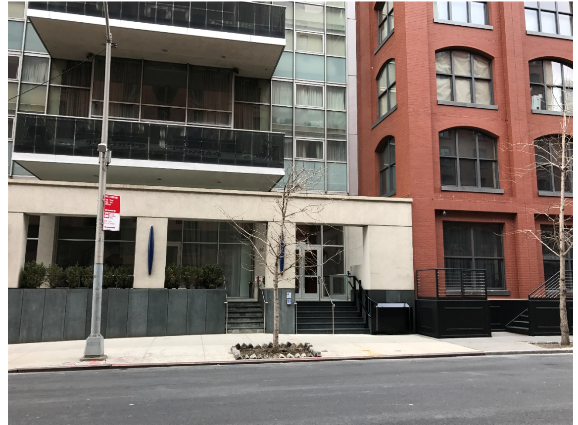
Residential Building Elevated to DFE – 3' above grade
