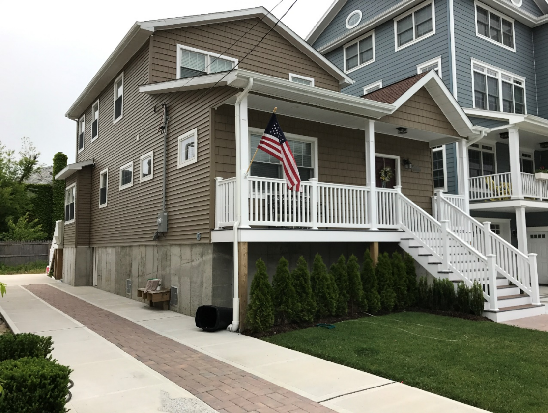
Residential Building Elevated to DFE
