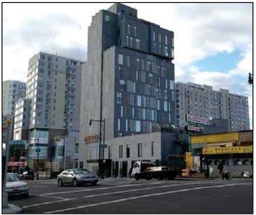
Parc Hotel - 2014 (12-story hotel) Image: NYC DCP
