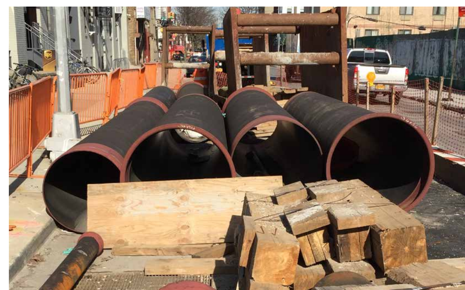
High-level storm sewer installation
