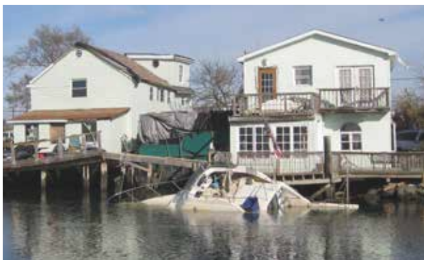
Houses damaged by Hurricane Sandy in Ramblersville, Hamilton Beach
