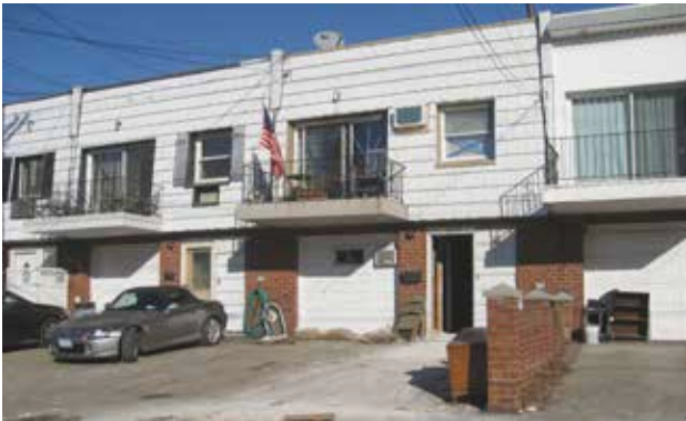
Attached housing in R3-2 district in Old Howard Beach
