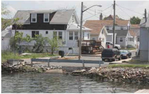
Low-lying street end at Hawtree Basin in Hamilton Beach
