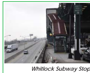
Whitlock Subway Stop
