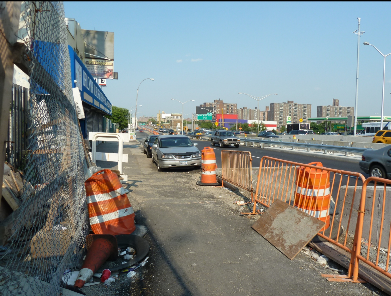
View sidewalk adjacent to U-Haul site
