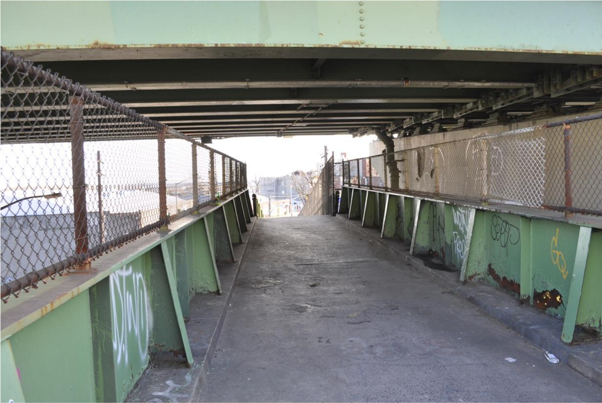
View from bridge under Bruckner Expressway
