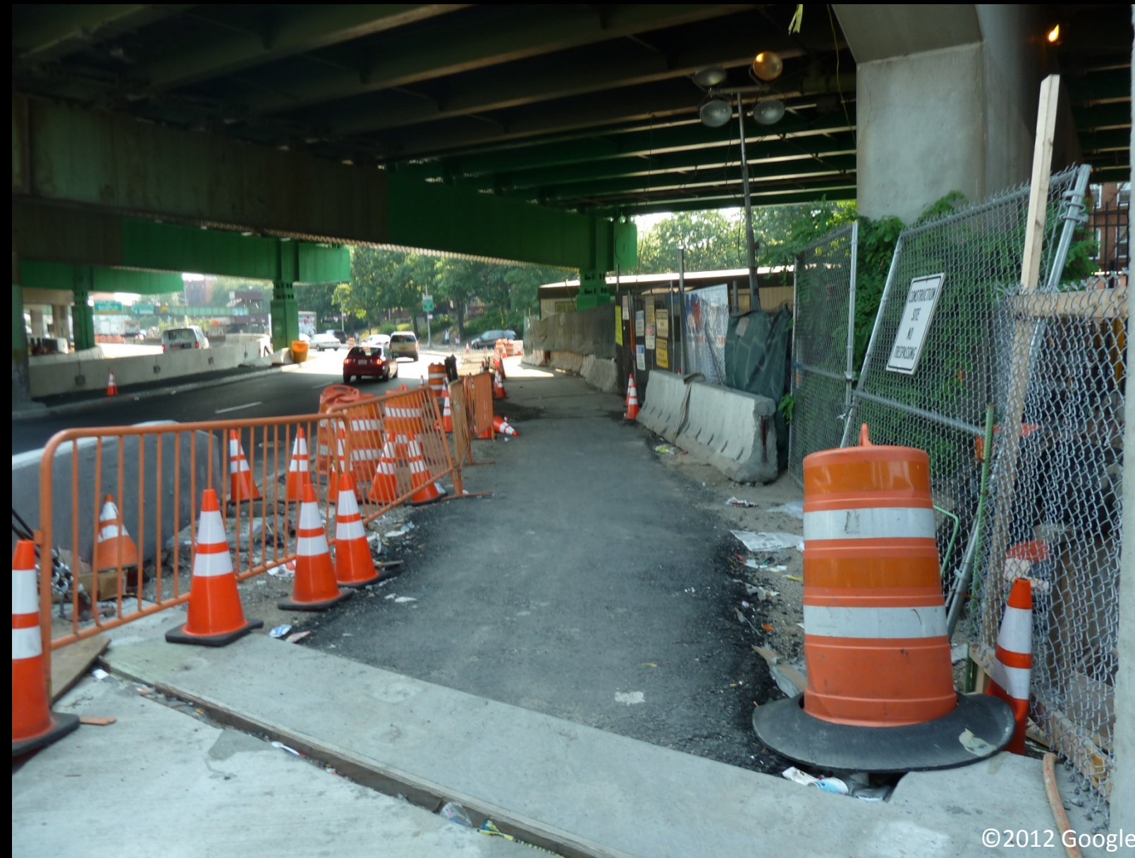
View sidewalk under Bruckner/Sheridan Expressway
