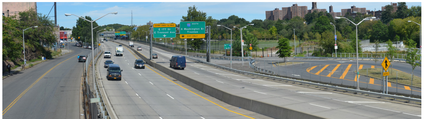
View of the Sheridan Expressway looking north. The southern entrance to Starlight Park is to the right.
