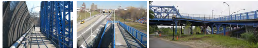
174th St Pedestrian Bridge Entrance
