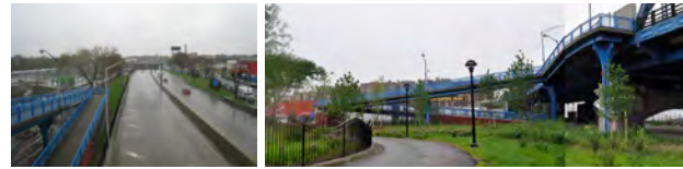
174th St Pedestrian Bridge Entrance
