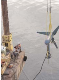
Verdant Power installing tidal turbine in East River
