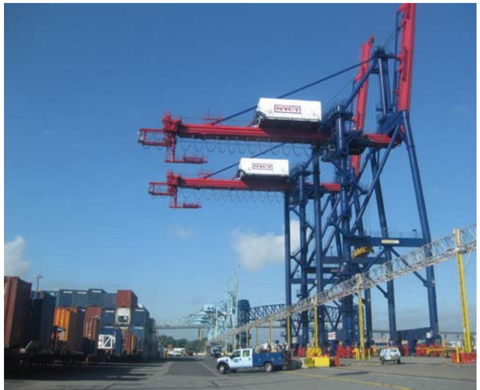
New York Container Terminal on Staten Island.
