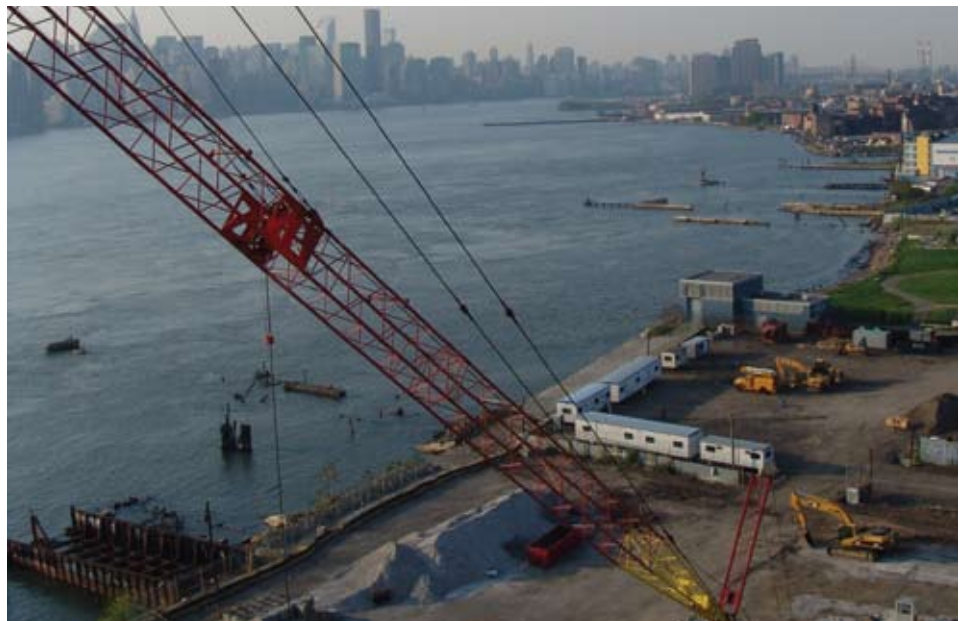
Redevelopment under way on the Williamsburg waterfront.
