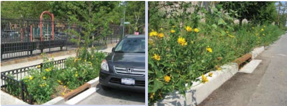
An enhanced tree pit, left, and swale, right, manage stormwater efficiently and also green neighborhoods.
