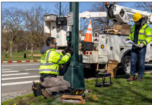
Above: A DOT employee installs an APS pushbutton. Right: A person who is blind uses an APS pushbutton before entering a crosswalk.
