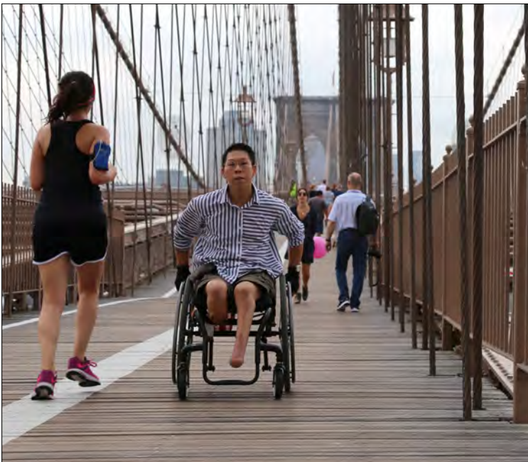
Brooklyn Bridge pedestrian path
