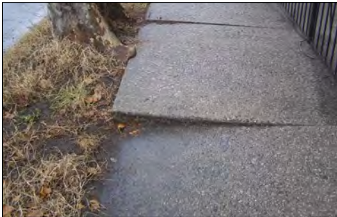
Left: Example of uneven surfaces along a sidewalk. Right: Sidewalk improvements remove obstacles for people with disabilities.
