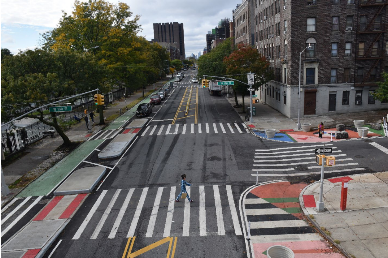
Amsterdam Avenue at W. 190 Street, Manhattan: asphalt art mural, two-way protected bicycle lane, bus boarding island, pedestrian safety island, ADA-accessible pedestrian ramp upgrades, speed cushion, kwik curb painted curb extensions adjacent to George Washington Educational Campus
