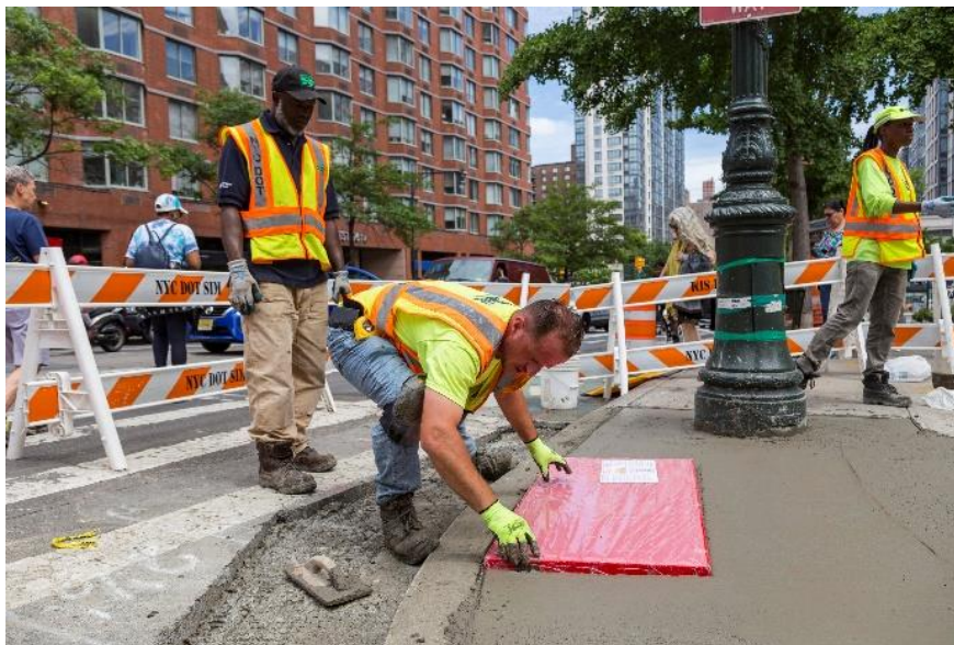
Accessible Pedestrian Signal and Pedestrian Ramp Installations
